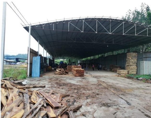
(f) a second roof for the teak sawnwood facility
