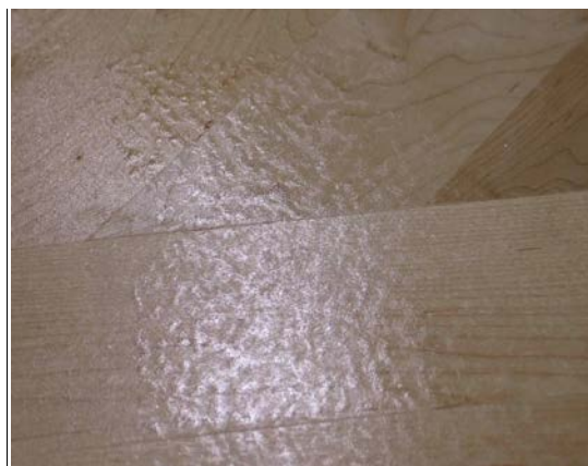
Figure 19: Orange peel (reproduced from http://hardwoodfloorsmag.com/forum/topic25-what-causes-this-finish-problem.aspx )
