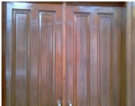
Figure 20: Blushing problem (reproduced from http://www.wisnofurniturefinishing.com/2010/04/blushing-problem-in-furniture-finishing.html )
